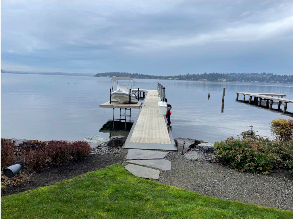
Photo 1 - Existing conditions looking waterward.
