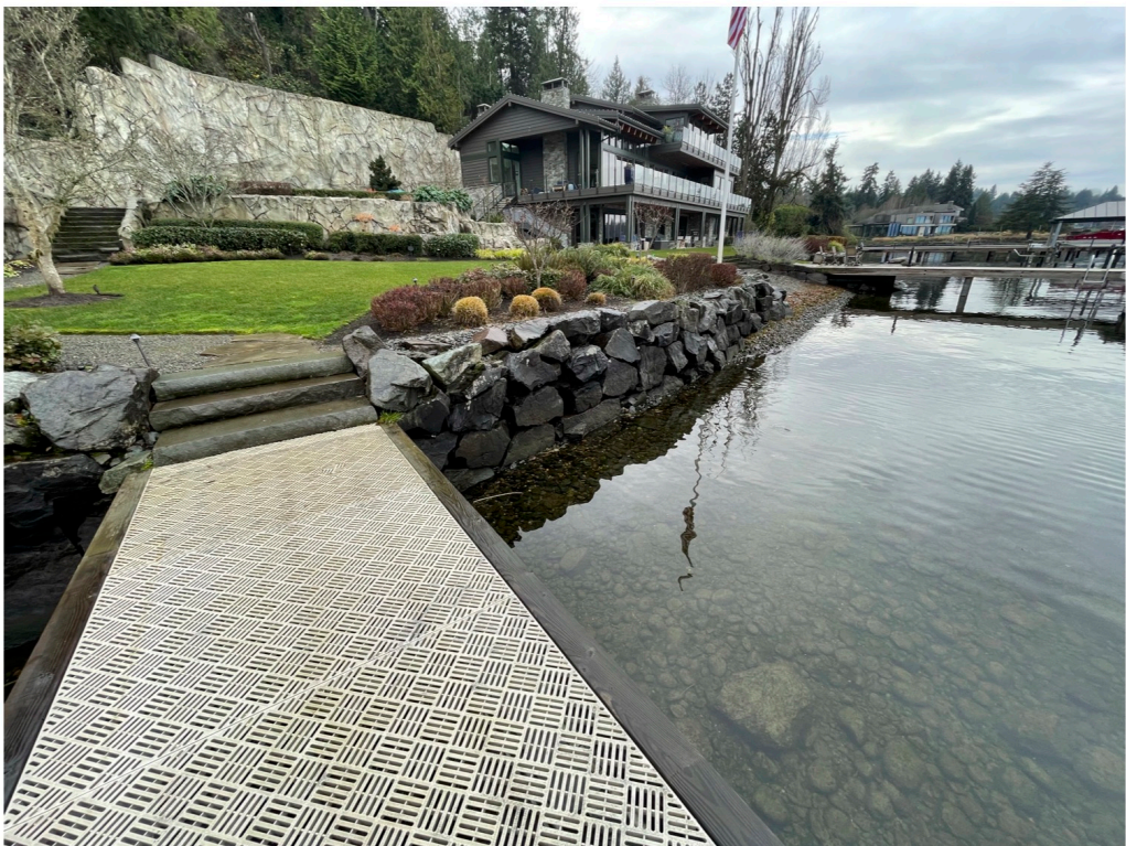
Photo 4 - Shoreline conditions west of the dock.
